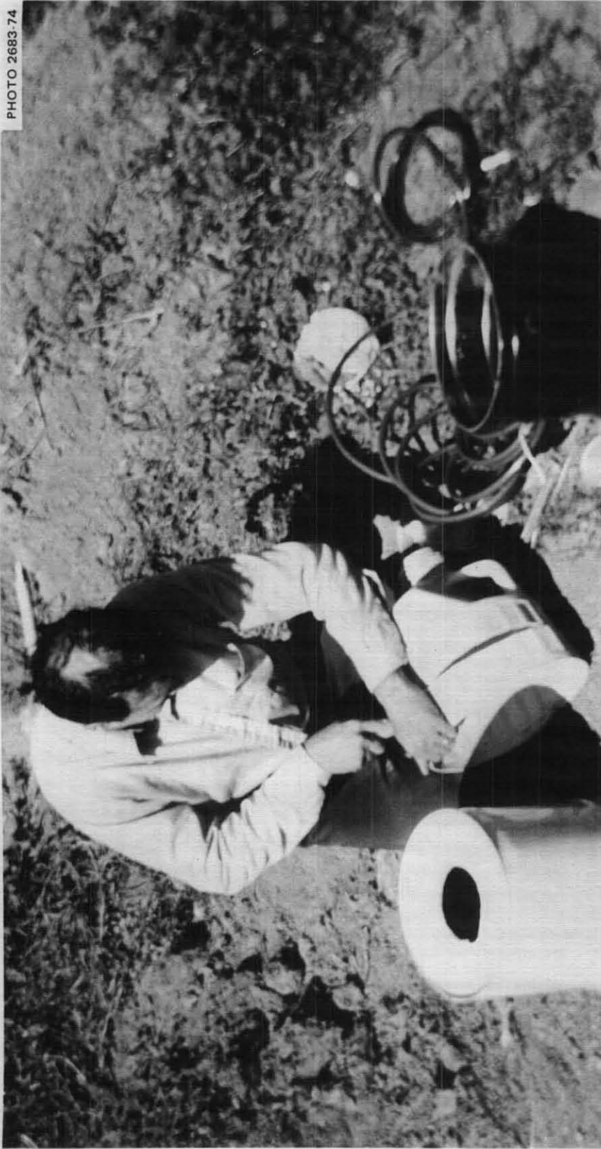
Fig. 4.26. Using a sharp knife to cut off the lower part of the 5-gallon plastic water jug, in order to make the bowl of the toilet. The bottom of the 5-gallon can shown on the right was cut out so that when this can was used to form the bottom of the 10-gallon vented space provided for the wastes, the liquid fraction could run into permeable earth or sand below.
